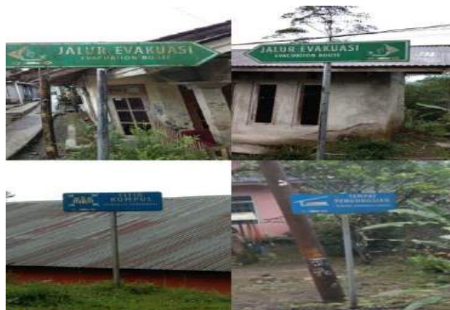
Picture 2. Evacuation Route Sign Source: Research Documentation, 2021
