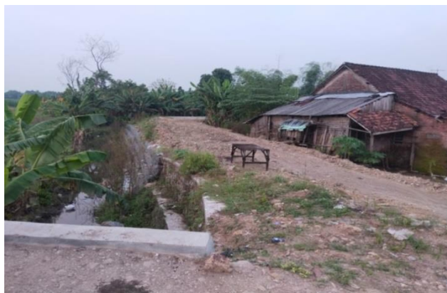
Figure 6. The embankment of Banyulegi Village that has been completely elevated
