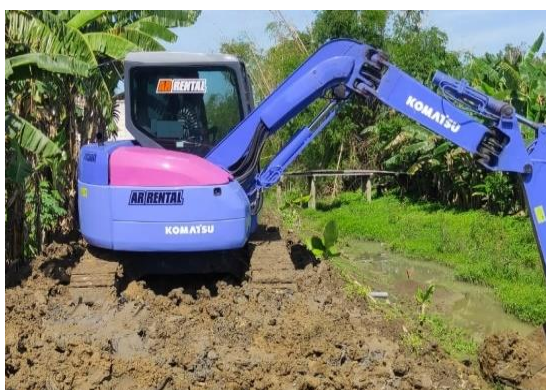
Figure 5. The process of elevating the embankment in Banyulegi Village
